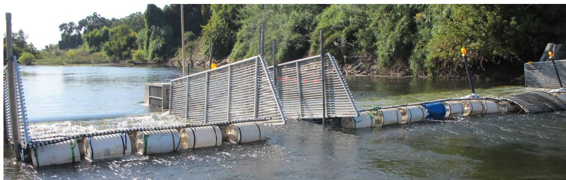
Figure 2. Photograph of the weir with sealed plastic barrels used for additional flotation.
