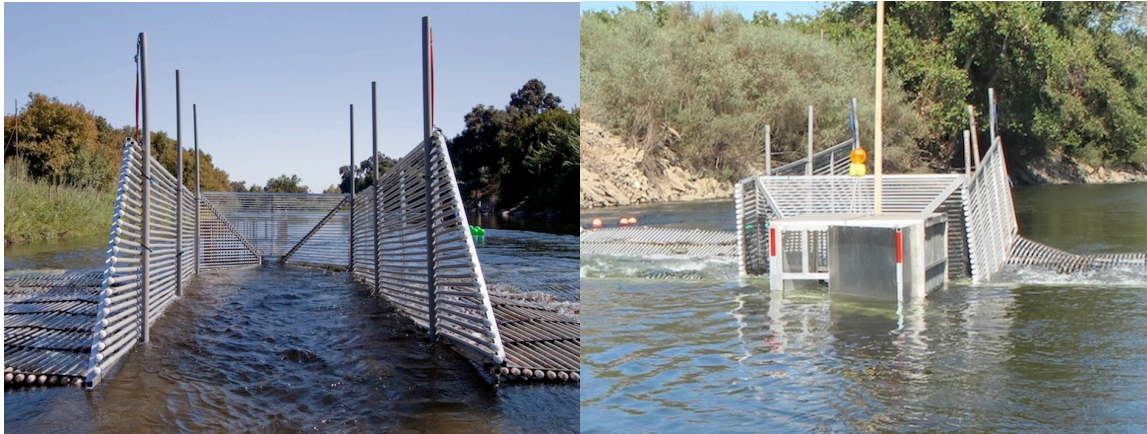
Figure 4. Left: Downstream photo of the fyke that contains Vaki system. Right: Upstream side of livebox where fish migrating upstream of the weir exit the Vaki system.
